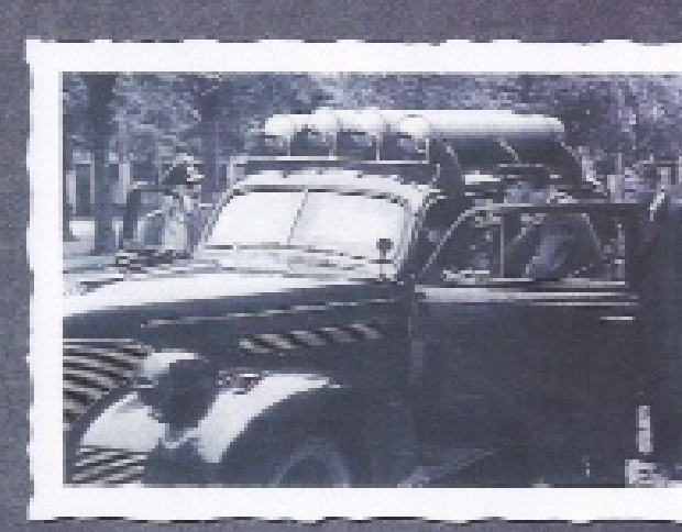
Occupation: German officers inspect a '39 Chevrolet modified to run on compressed gas.
